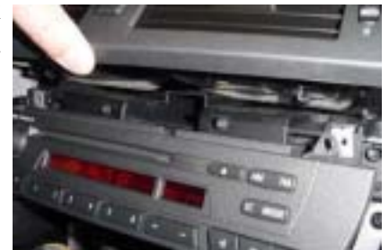
Removal of air vent assembly
